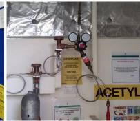
The VIQ makes no reference to the flashback arresters requiring periodic maintenance. However, the same publication (British Compressed Gases Association Code of Practice CP7) states Flame arrestors and their integral cut off valves should be replaced with a new or refurbished unit 5 years from the date of manufacturer or as per manufacturers recommendations.
