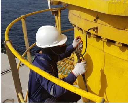
containing Molybdenum Polysulphide (MS2) can cause the bearings to slide rather than roll in some slewing ring types, increasing the wear rate. Excessive old grease emanating from sealing rings must be removed and disposed of in line with regulatory requirements to prevent it from falling onto the main deck or external crane ladders, creating a slip hazard.
