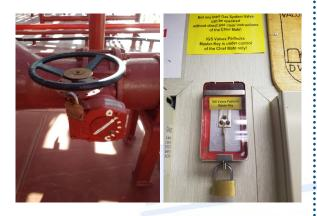
Here we have the padlocks protected so that they can be opened easily and a clear statement in the CCR as to the level of authority for the control of these valves.
